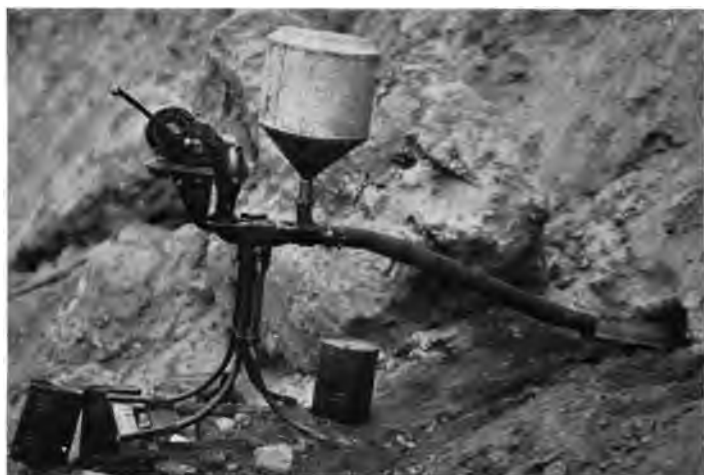
Fig. 3. Device for Blowing Powder into Holes for Blasting.*
